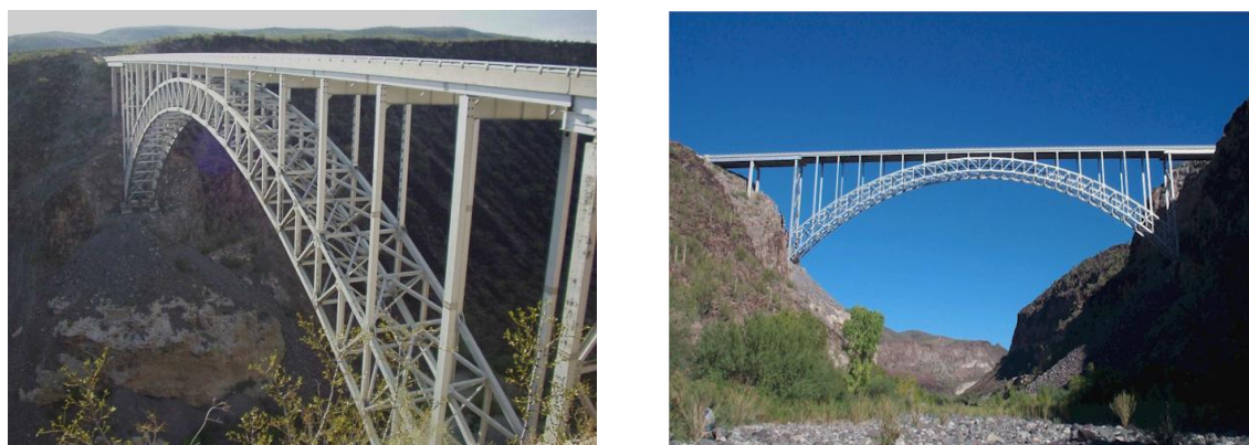
Figure 1. Burro Creek Bridge
