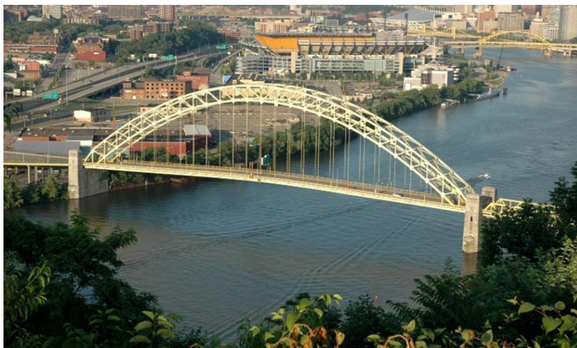
Figure 5. The West End-North Side Bridge
