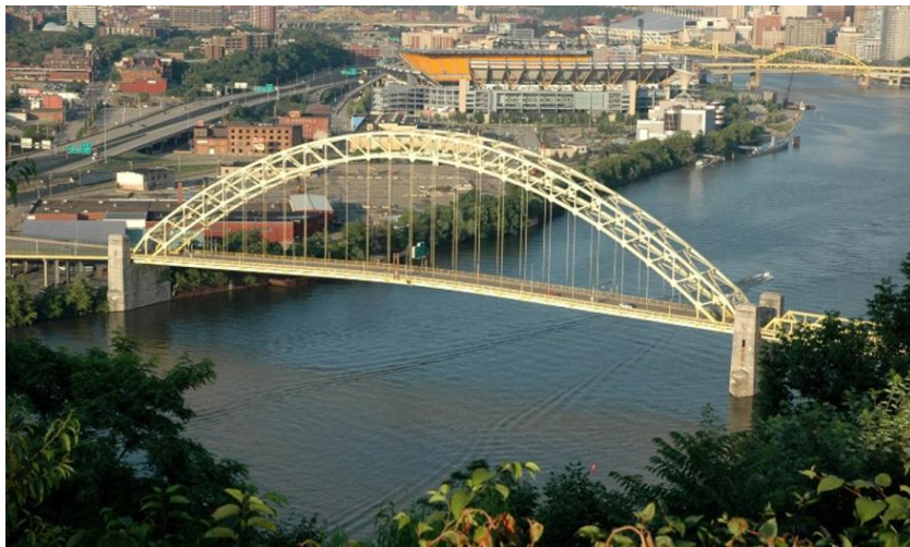
Figure 5. The West End-North Side Bridge
